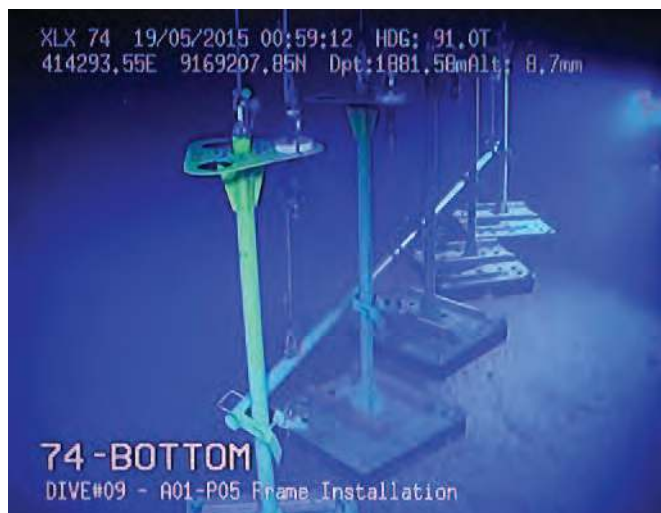
Ahead of the offshore campaign, the proposed location for each Compatt was carefully analysed. This verified that there was clear line of sight between each transponder so that they could reliably range to each other.
